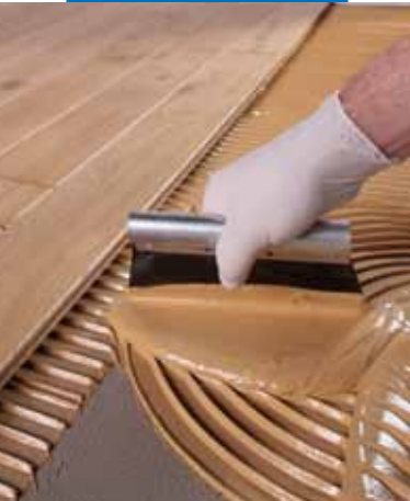
Spreading Ultrabond P990 1K
